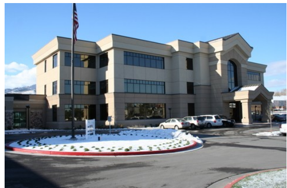
Mountain View Hospital's Medical Office Building
